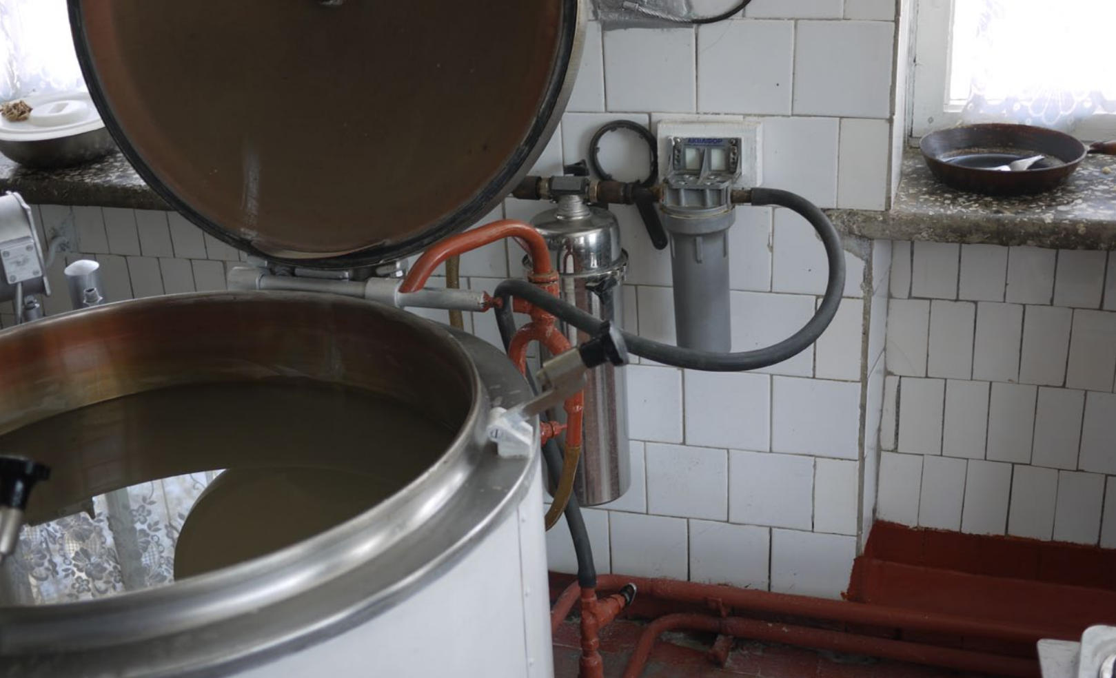
Water filters, which are supposed to last for three years, have to be changed after just nine months in Mailuu-Suu, Kyrgyzstan, because of the high level of contamination Photo credit: Blacksmith Institute for a Pure Earth
