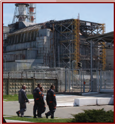
Construction workers at the Chernobyl Nuclear Power Plant. (Source: GCI).
